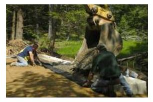
prepare the steel bridge frame donated from Boston's Big Dig project. Mark transported the structure and set it onto the abutments using his large excavator plus an extension arm.
