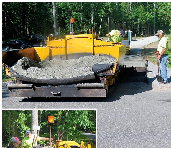
Top coat for new section of trail at Mill Street, Holden
