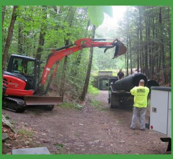
Sometimes major maintenance is needed. Here new culvert pipes are readied for installation on the Charnock Hill Rd. to Miles Rd. section of the MCRT in Rutland. In 2022 we also contracted full restoration of the ditches here. In 2023 we'll resurface portions of this well-traveled section.
